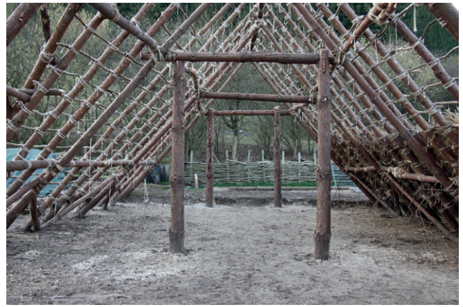
Interior of Horton House 2 with A-frame construction at Butser Ancient Farm. © Trevor Creighton 2019
