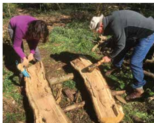
Cutting mortises in the split log
